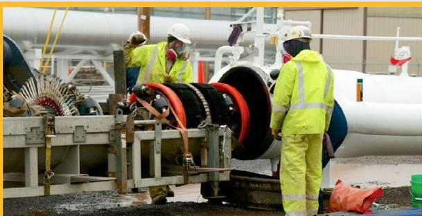
Internal pipeline inspection is part of pipeline maintenance and is performed regularly to check for cracks, dents and corrosion. In-line inspection devices sometimes referred to as "Smart Pigs" use sophisticated technology to assess the condition of the pipe electronically, allowing precise analysis through data collection. The data is then reviewed and helps determine if there is a need to excavate a section of the pipeline for further inspection.
