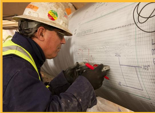
Typically, the area of the excavation is stripped of topsoil, which is stored separately from the subsoil. After the pipeline is excavated, the pipe coating is removed so the pipeline can be inspected. If needed, any repairs will be made and the pipeline (and coating) will be restored to proper condition.
